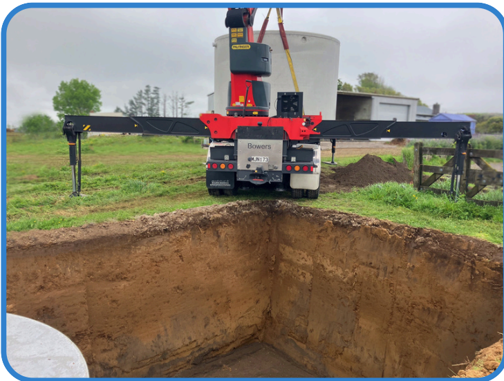
Example of the correct truck position for unloading into the prepared site.
