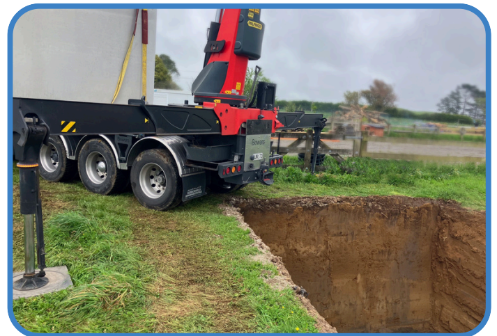
Side angle of the of the correct truck position for unloading into the prepared site.
