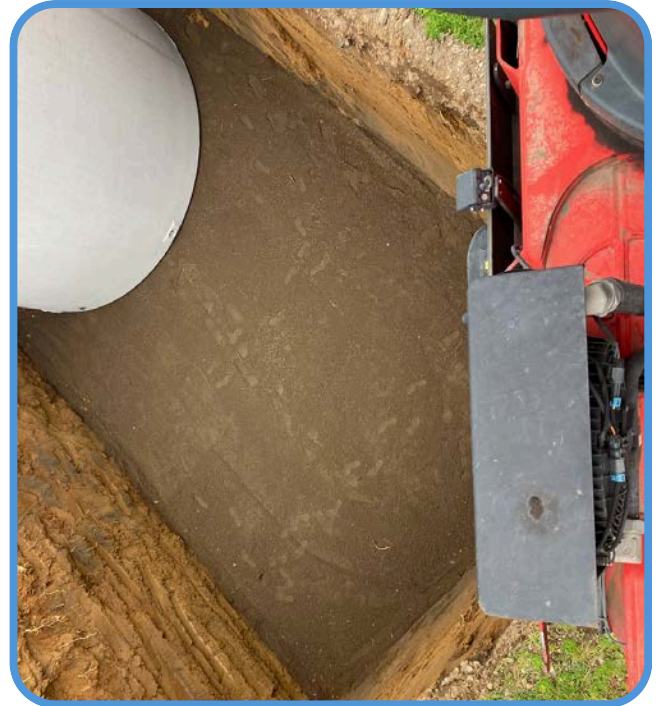
Birds eye view example of correct truck positioning.
