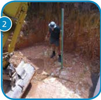
2 The excavated hole should be square. The final size should be 4.2m x 4.2m x 3.125m deep. This allows for placement of 100mm compacted hard fill and 75mm granular fines on base of excavation, plus the overall height of tank which is 2950mm
