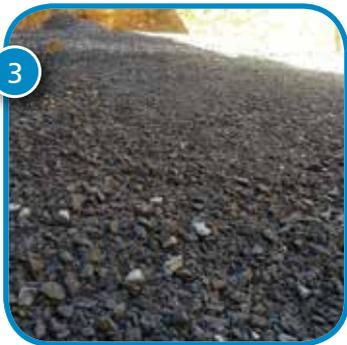
3 Ideally hard fill added and compact to a depth of 100mm thick
