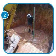
The excavated hole should be square. The final hole size should be 5m x 5m for 4.3m(extended base) diameter effluent tanks and 4m x 4m for the 3.74m (std base) diameter tanks.
